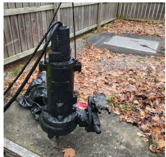
7th Street pump annual lift station inspection.
