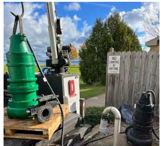
Main lift station new pump install.
