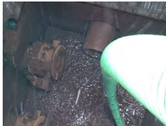
Annual plant wet well chamber cleanings.
