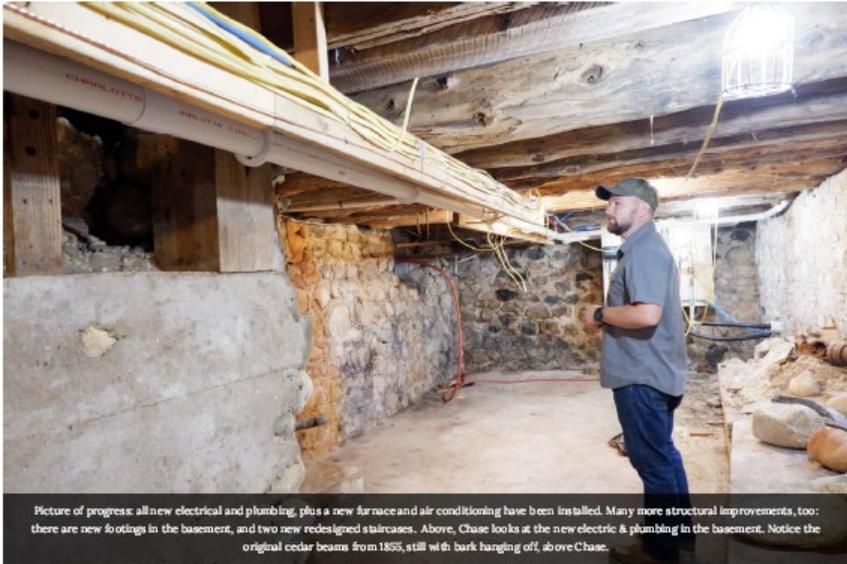
Picture of progress: all new electrical and plumbing, plus a new furnace and air conditioning have been installed. Many more structural improvements, too: there are new footings in the basement, and two new redesigned staircases. Above, Chase looks at the new electric & plumbing in the basement. Notice the original cedar beams from 1855, still with bark hanging off, above Chase.
