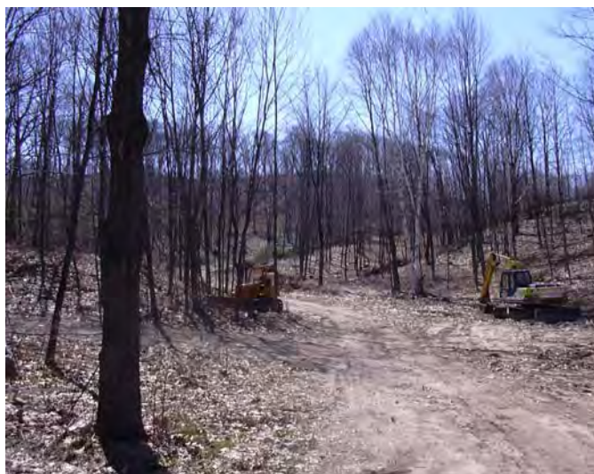
New road construction in Leland Township
