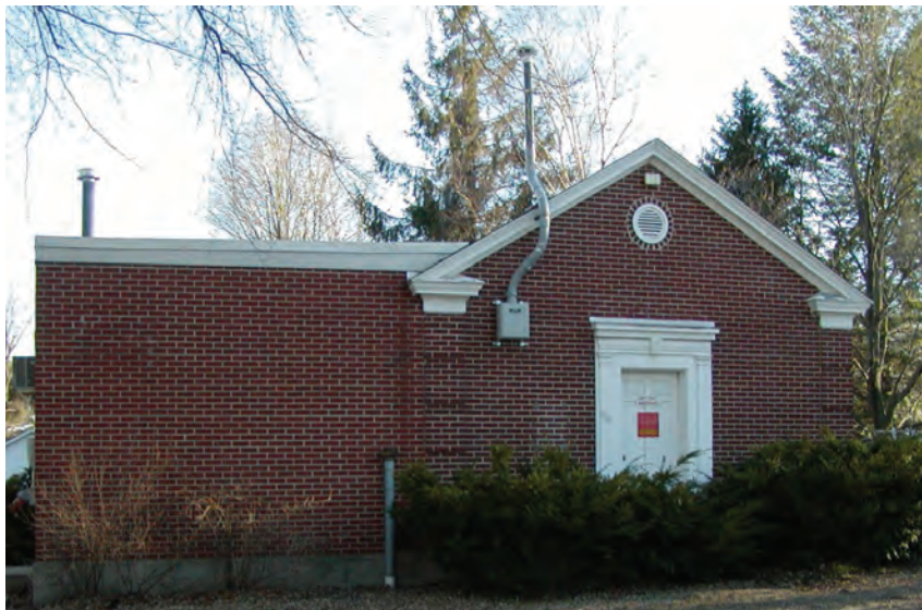
SBC Ameritech building in Northport
