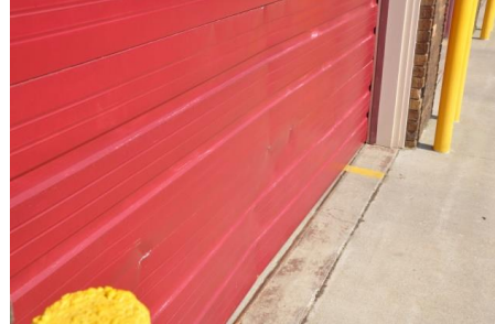
FIGURE 20 - EXTERIOR VIEW OF BAY DOOR
