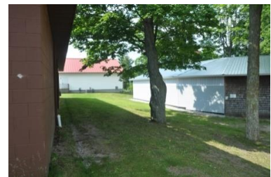
FIGURE 29 - REAR VIEW OF STATION 2
