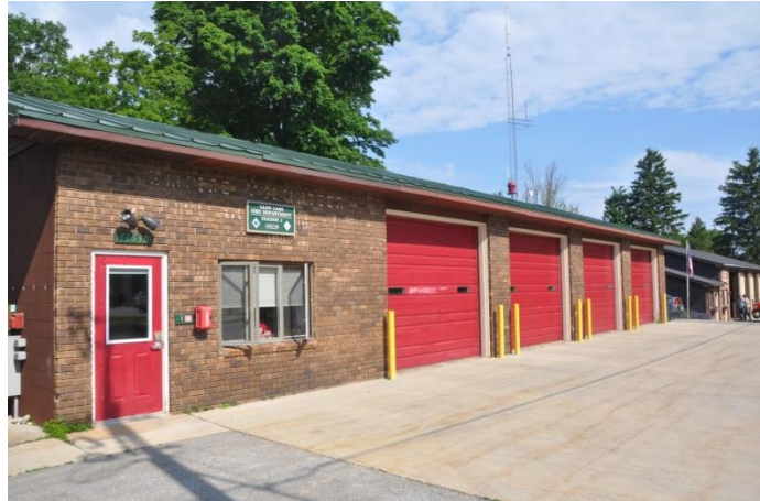
FIGURE 26 - EXTERIOR VIEW OF STATION 2
