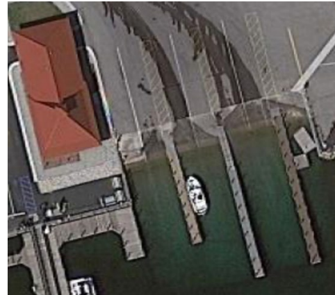
Figure 7 - Launch Ramp Area
