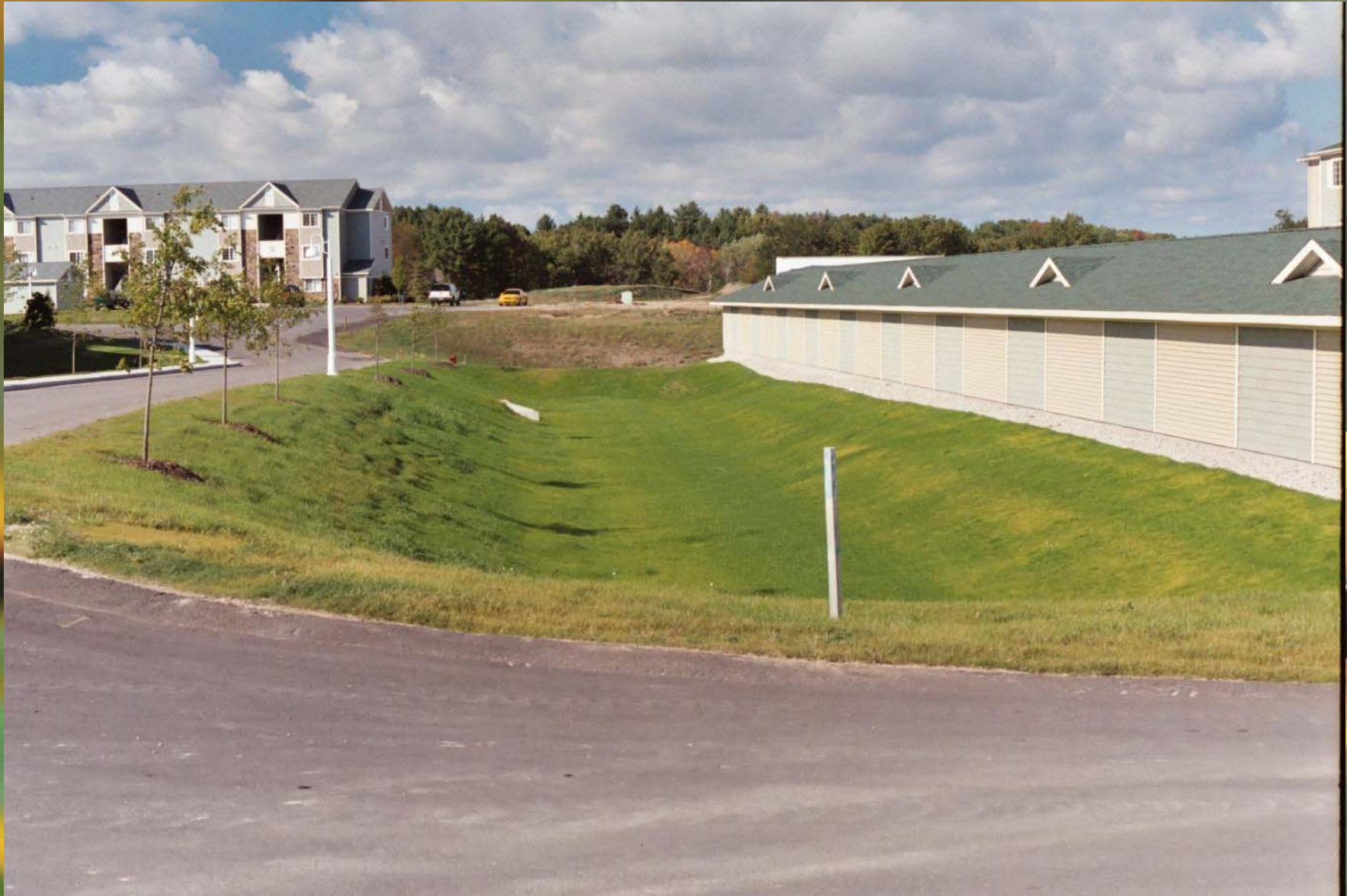
Traditional detention pond
