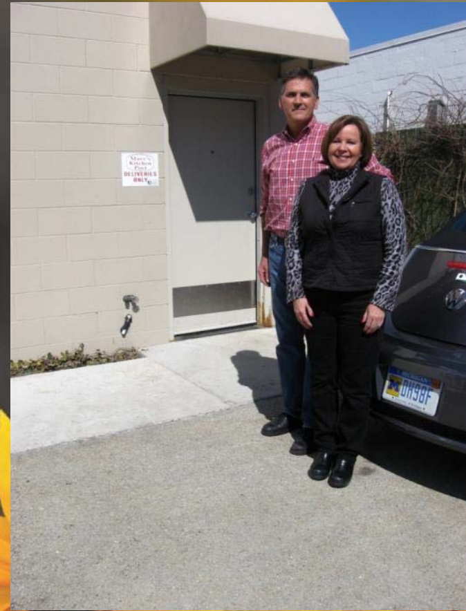
Pervious concrete at Mary's Kitchen Port (TC)
