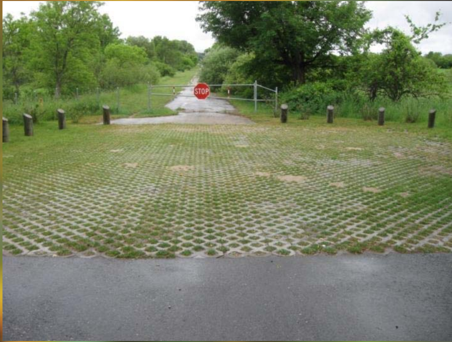
Pervious pavers at end of Elmwood Ave (TC)
