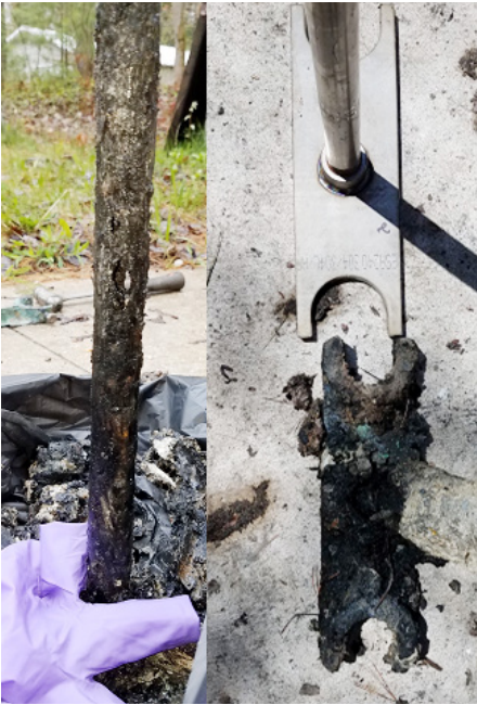
Old and new pump guide rails and bracket.
