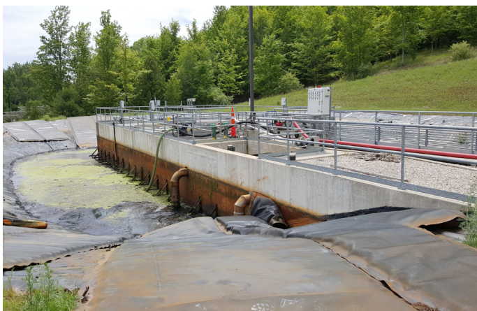
Settling basin cleaning.
