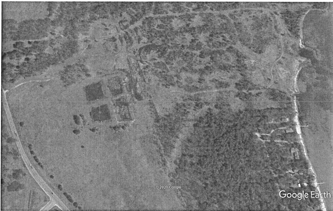
Figure 2. General perspective of the construction site. Date of image is 5/15/2018.
