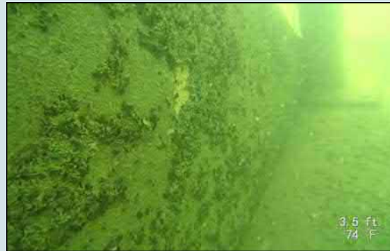
Leland Dam MI Dam ID.510 Leelanau County
