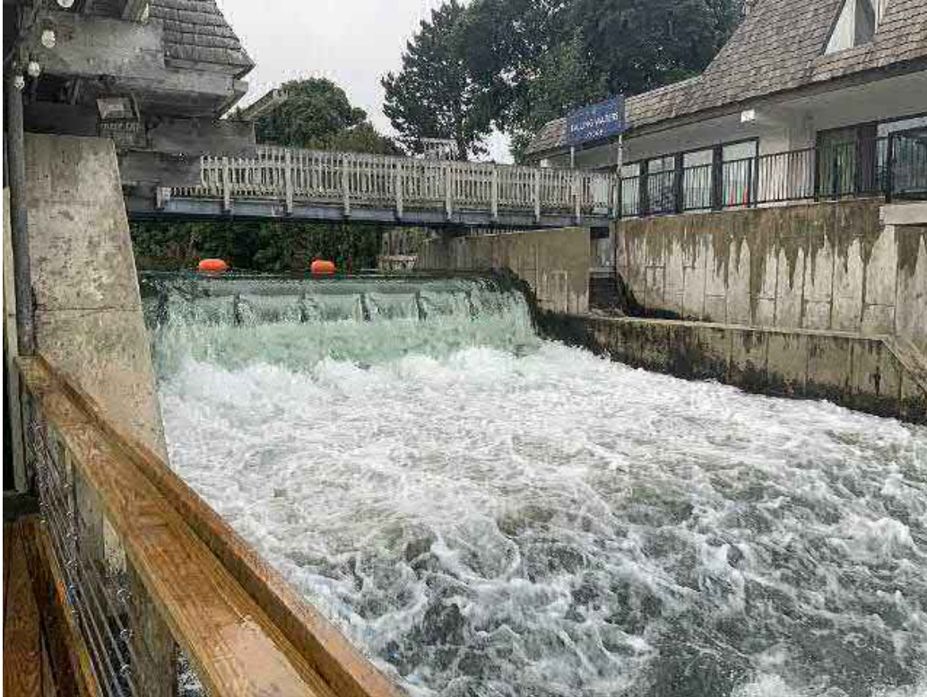
Looking south at downstream face of principal spillway (actuated weirs).
