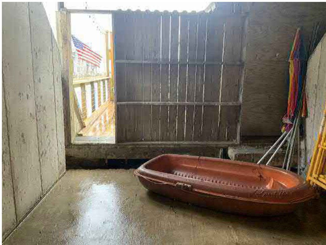
Looking downstream from just downstream of main door into hydraulics / control room.
