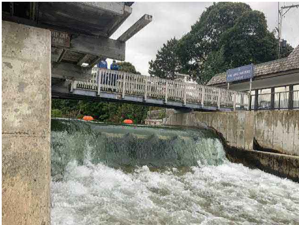
Looking southeast principal spillway (actuated weir gate).
