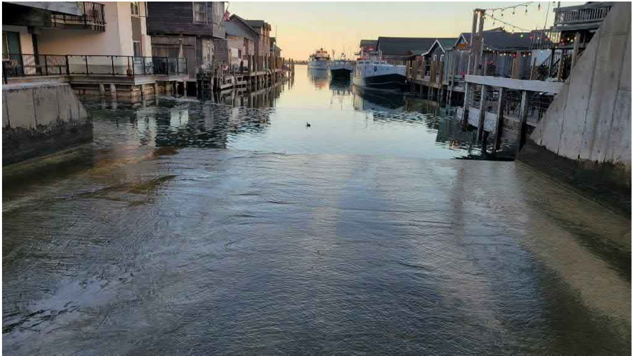
Looking Downstream from Hydraulic Gates within Primary Spillway
