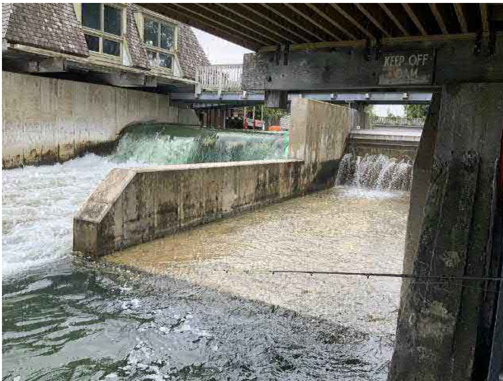
Looking east across downstream end of Bay #1 spillway.
