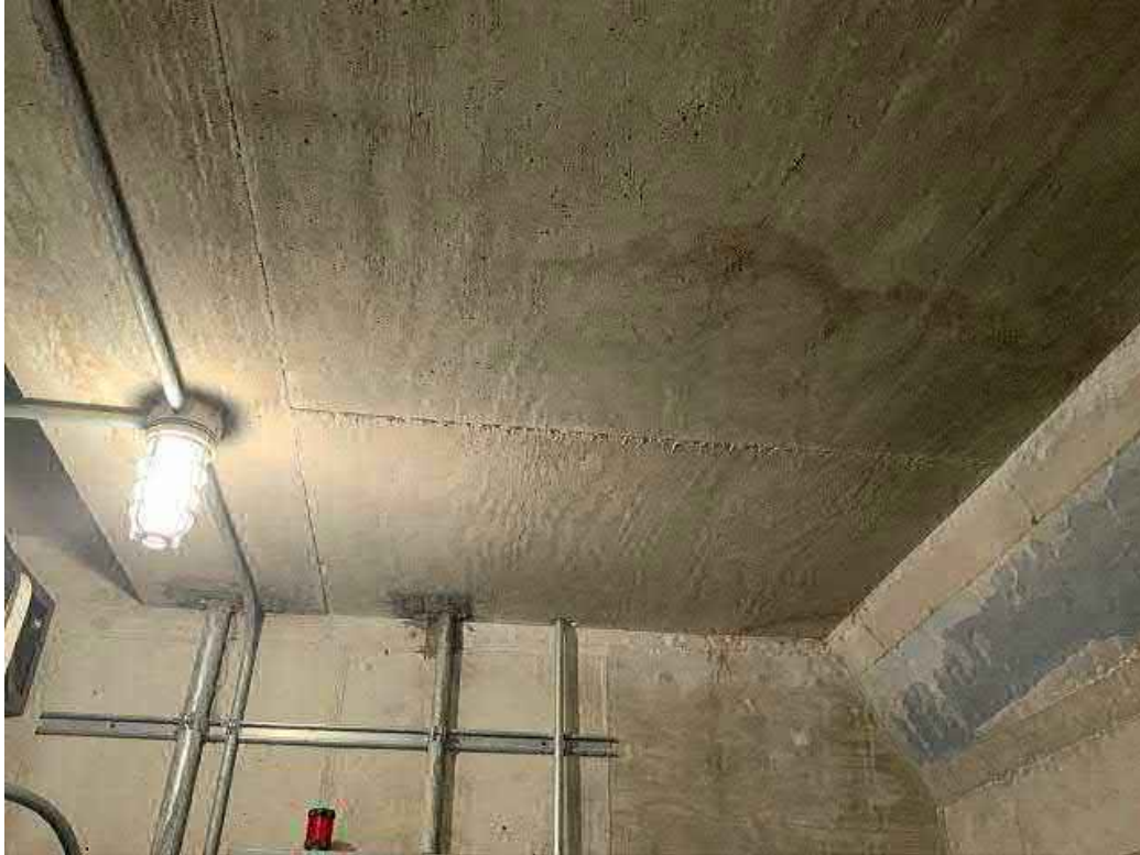
Looking northeast at ceiling of hydraulics / control room.
