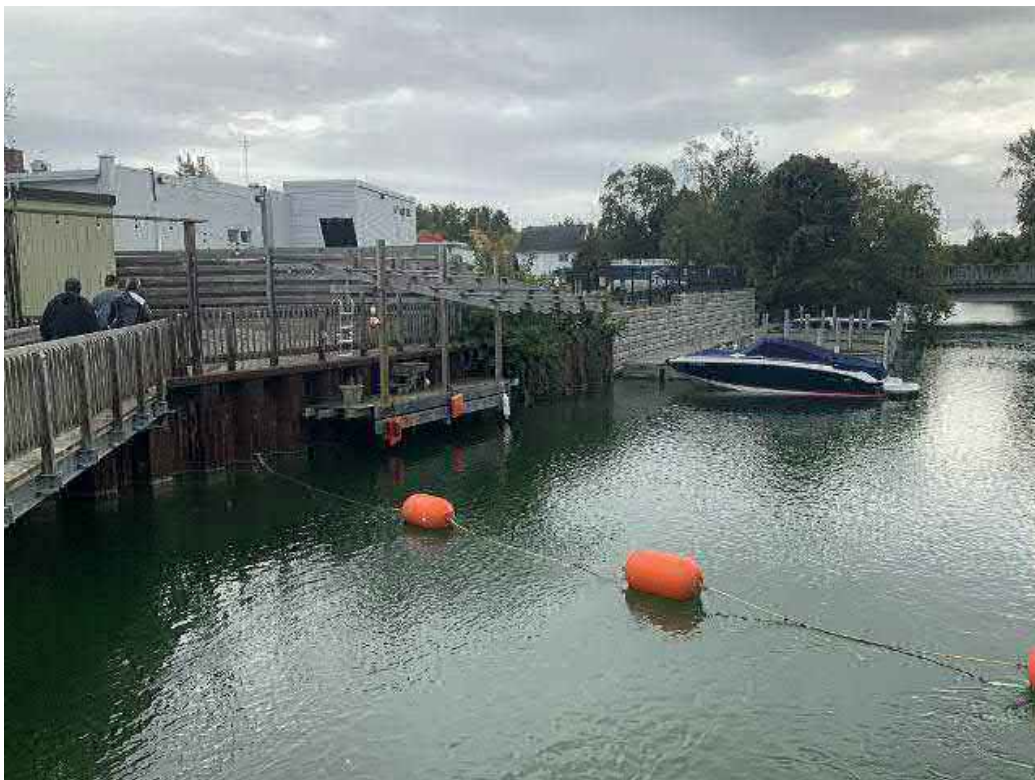
Looking east at upstream channel, warning buoys and walkway.
