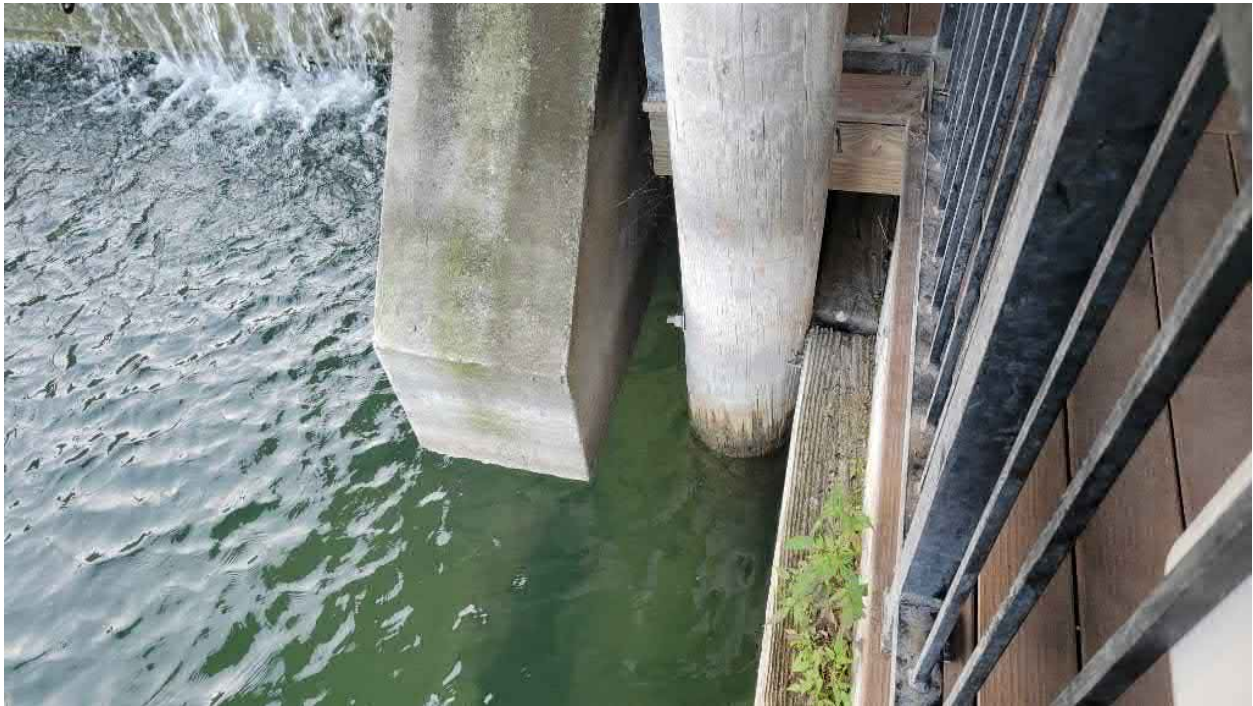
Pylon Behind Auxiliary Spillway Headwall
