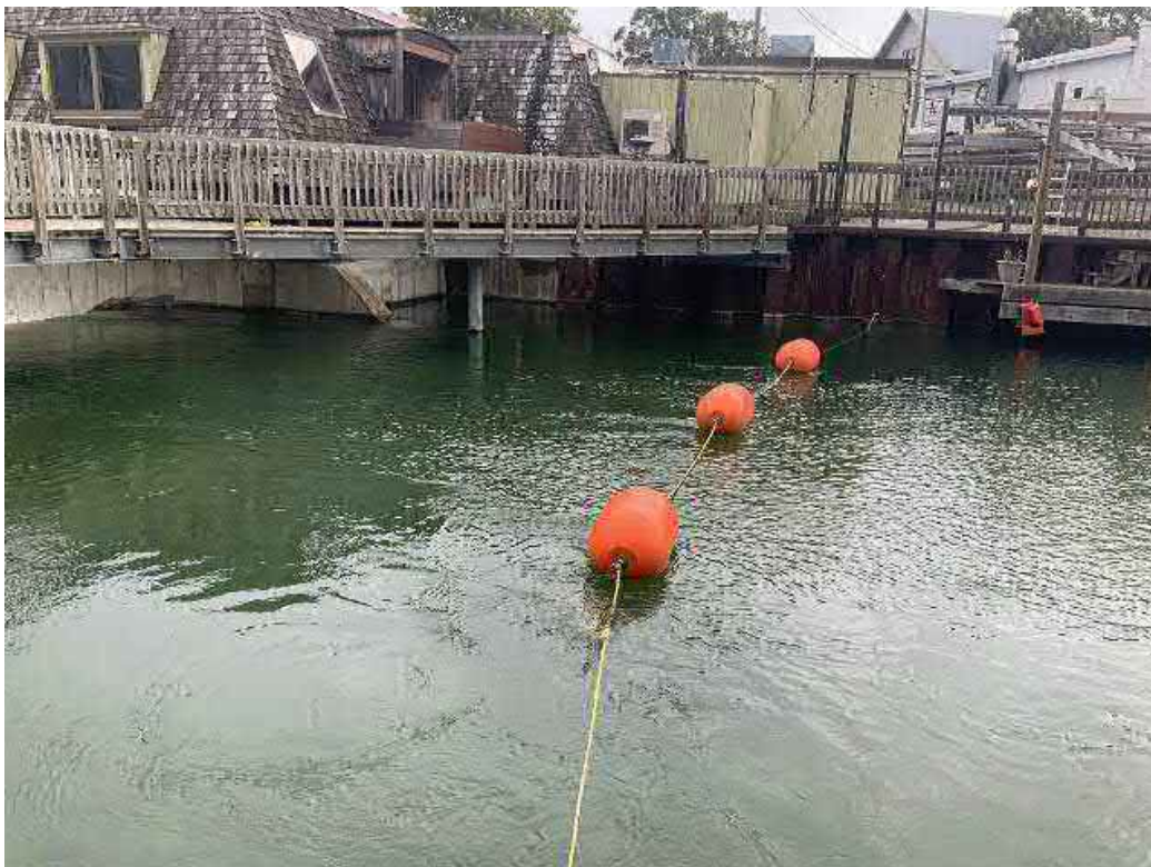
Looking northeast across upstream side of dam (warning buoys).
