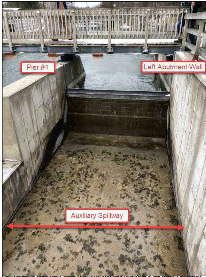
Looking Upstream at Auxiliary Spillway
