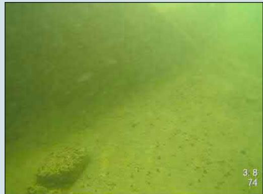
Pier #1 (upstream end)
