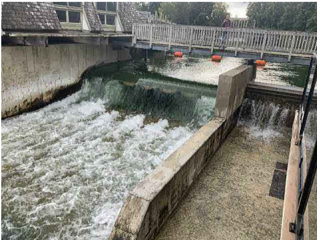
Looking southeast at Principal (former Bay #2 and #3) and fixed crest / stoplog (Bay #1) spillway.
