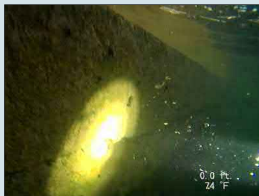
Downstream edge of spillway
