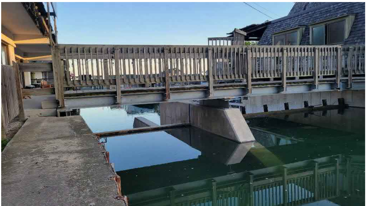
Catwalk above Dam to Access Auxiliary Spillway Boards
