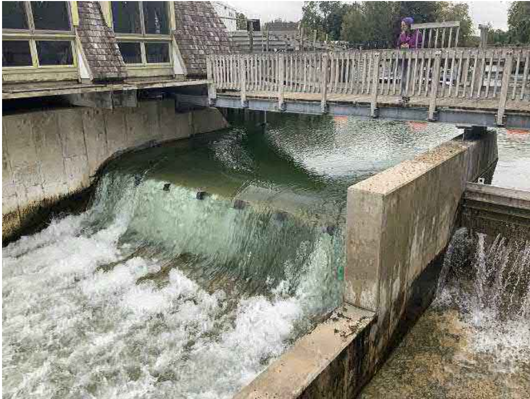
Looking east at principal spillway (actuated weir gate).
