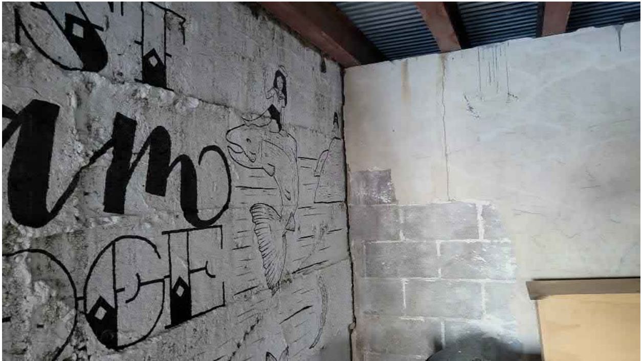
Left Abutment Wall and Wall Adjacent to Dam
