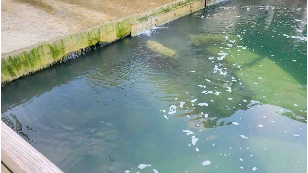
Spillway Observation While Gates are Closed
