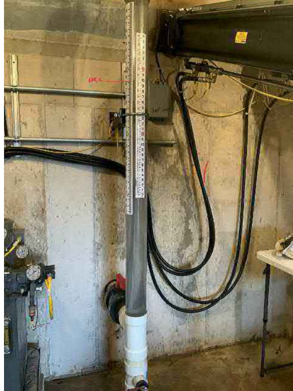
Water Level Gauge - reading 598.2' on date on inspection.
