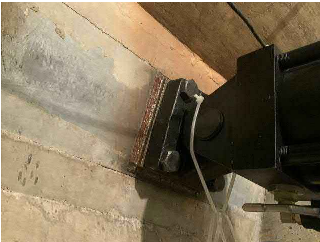
Hydraulic ram mounts to steel I-beam at ceiling / wall corner (typical of 2).
