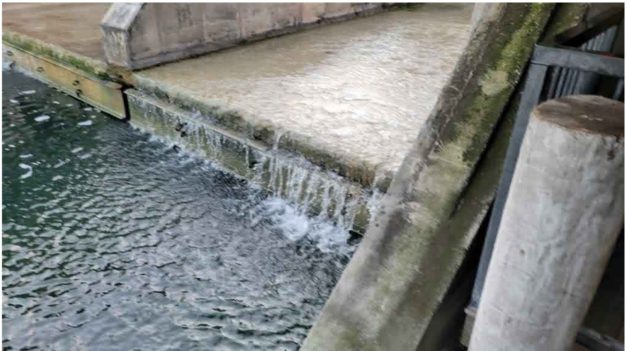
Downstream Face of Auxiliary Spillway
