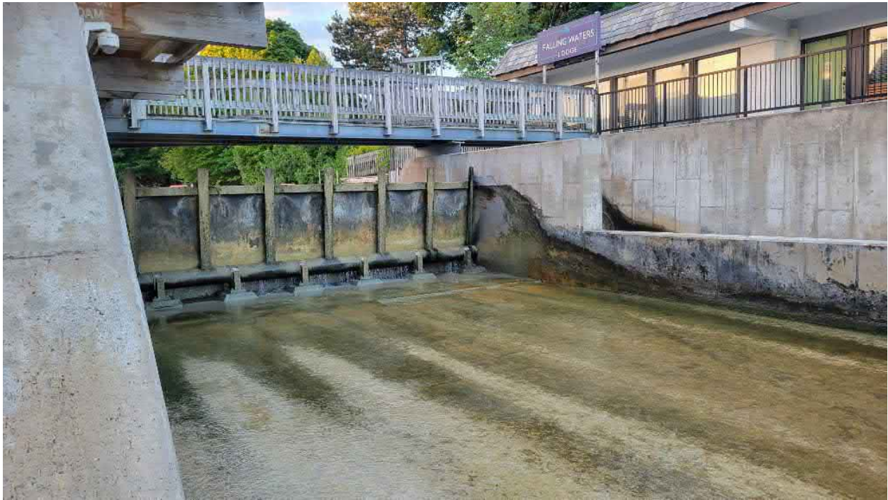
Downstream Face of Hydraulic Gates (Closed Position)
