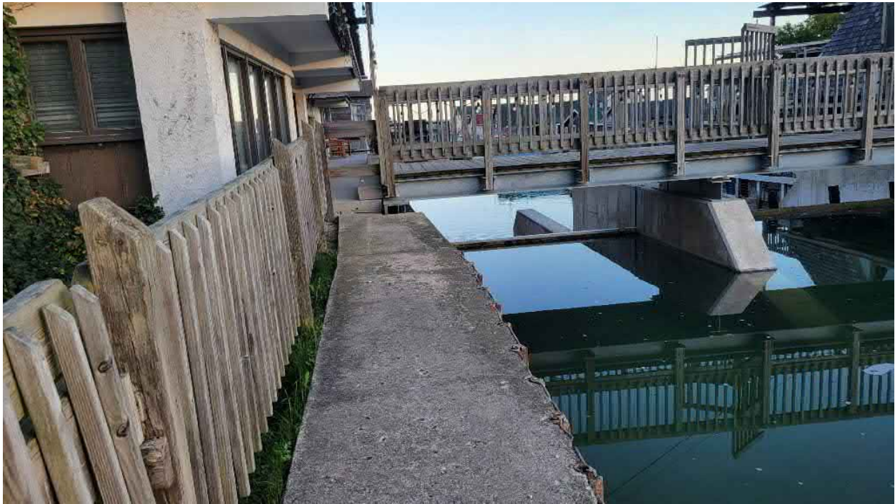
Left Abutment Wall
