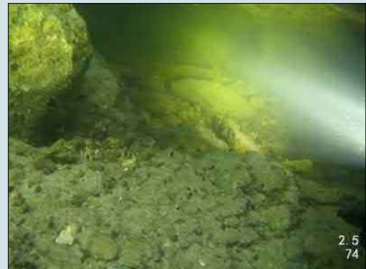
Cutoff wall and right abutment
