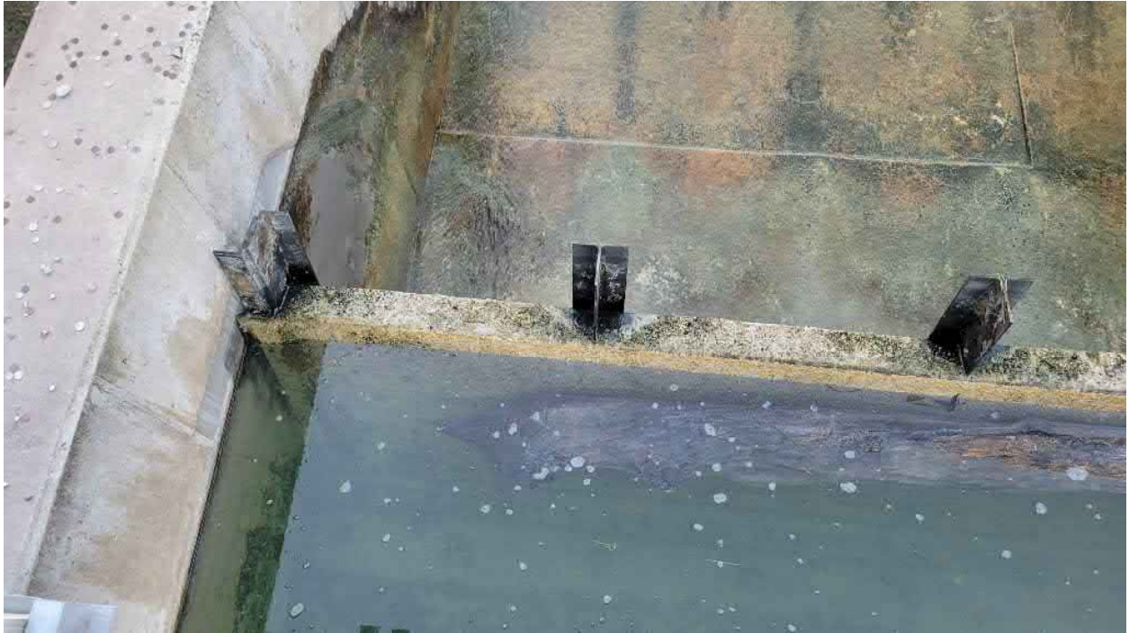
Closed Hydraulic Gate (Left Side)
