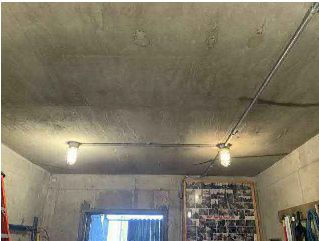
Looking northwest at ceiling within hydraulic / control room.
