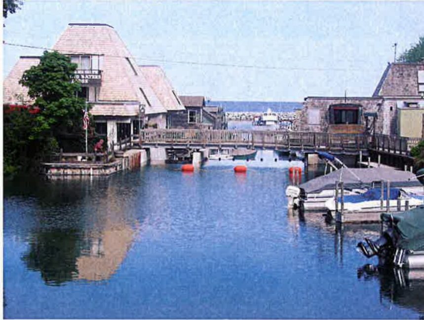
Photo 1. Upstream (US) view of Leland Dam spillway structure.
