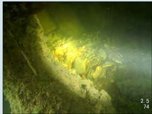
Left abutment (downstream end)
