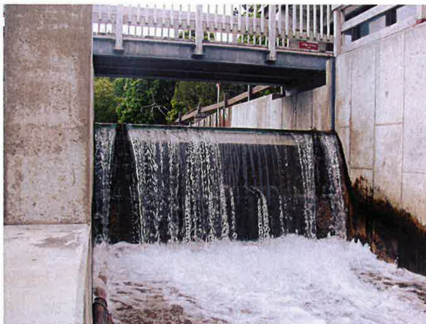
Photo 6. DS view of auxiliary stoplog spillway and access bridge.
