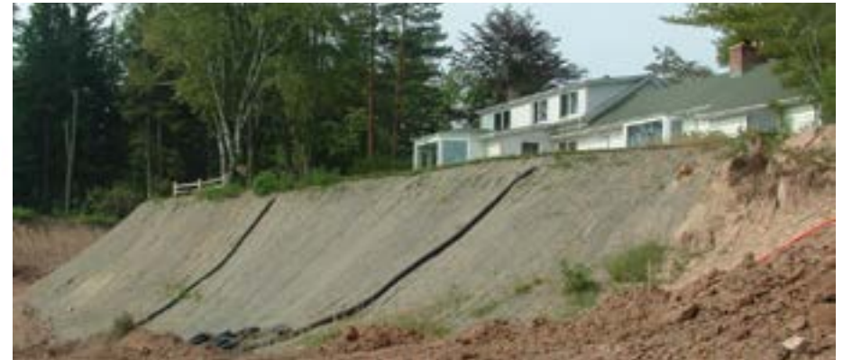
Figure 10: Terraced Bluff Stabilization Method
