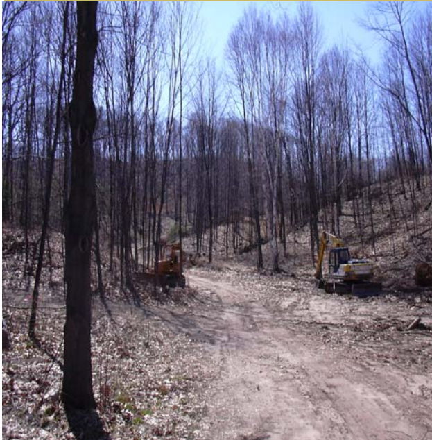
New road construction in Leland Township
