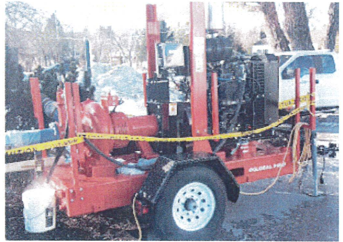
Main lift station bypass pumping.
