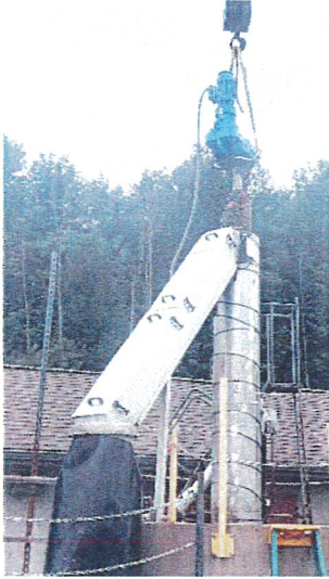
Fine screen auger removal by crane.
