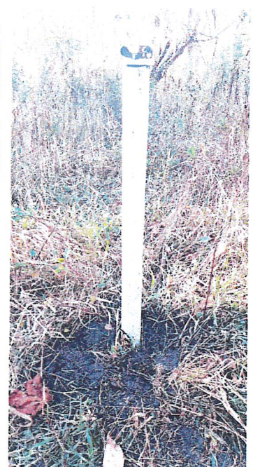
Repaired well casing pipe.
