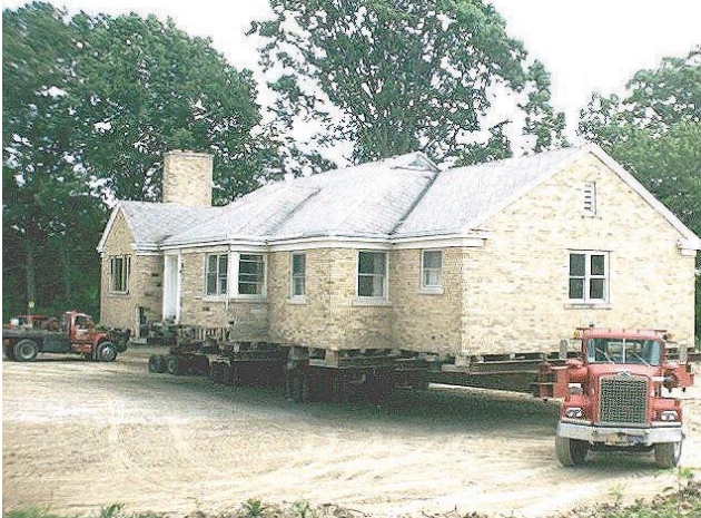
Relocating a house
