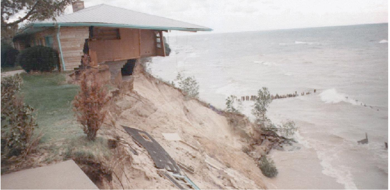
A house lost to erosion
