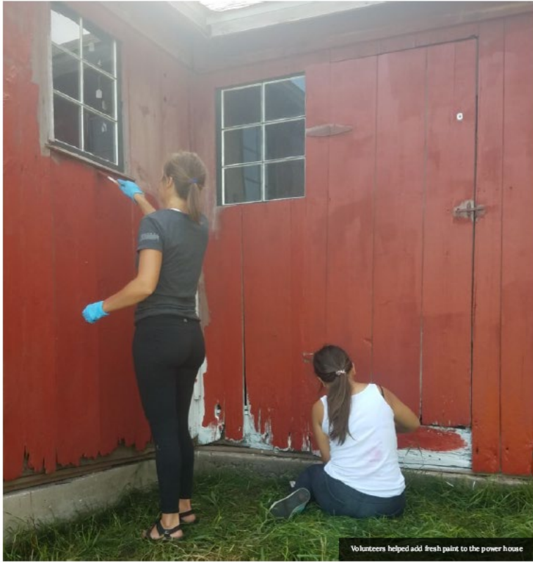
Volunteers helped add fresh paint to the power house
