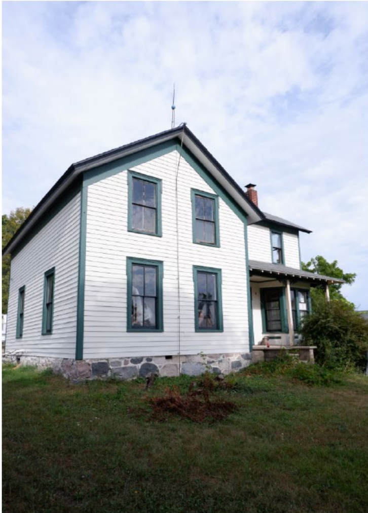
"The most visible change to the farmhouse so far is the new paint colors. "It was important to us to keep the original character of the house with tasteful updates," Chase says. "We chose historic paint colors with a traditional light primary color and dark trim (Ancient Ivory and Lafayette Green). We are also able to restore and keep the original wavy glass windows downstairs."
