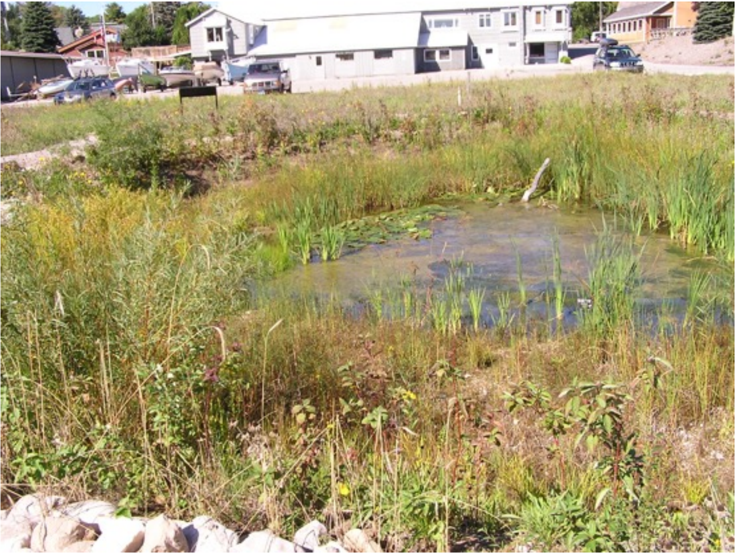
Year 2 - Deep basin of the innovative stormwater treatment system, ISEA Center, 100 Dame St., Suttons Bay, MI - Grobbel Environmental & Planning Associates design and construction.
