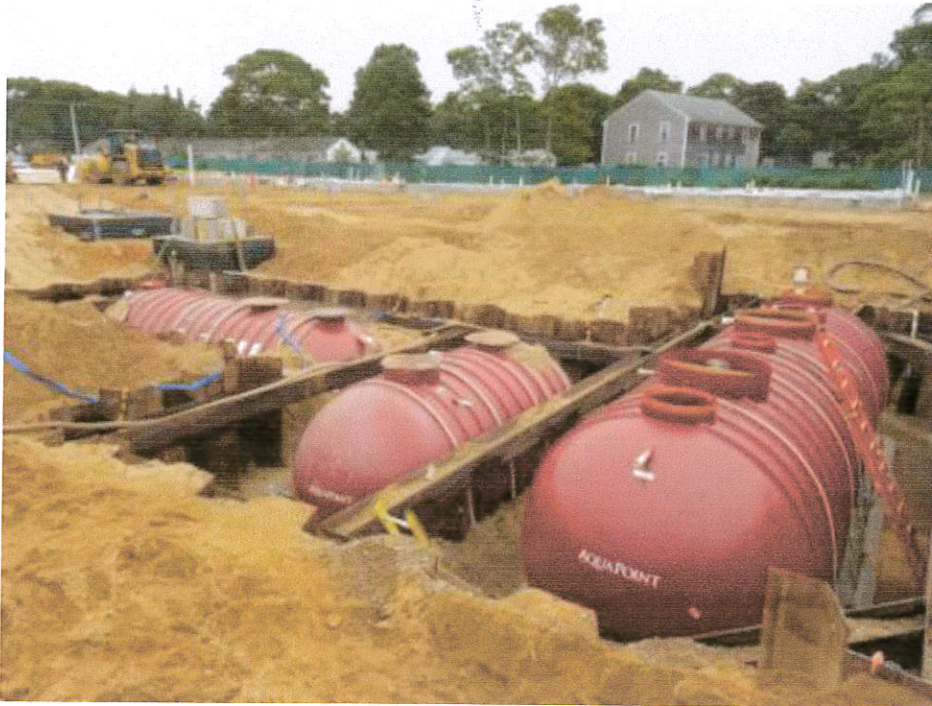
Typical underground tank installation
