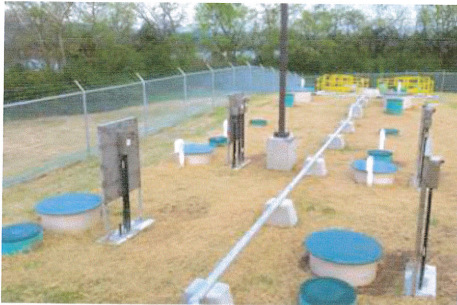
Typical access hatches after completion
