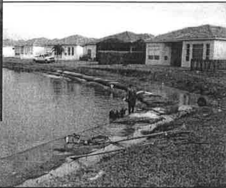
Geotube® LES™ being installed
