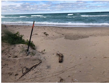
Labor Day Sep 7, 2020 Drain Plugged, Channel Covered
