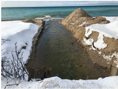
Outlet Drain Flowing to Lake Michigan
