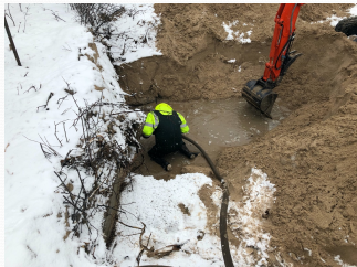
Clearing Culvert with Firehose Jan 23, 2020
