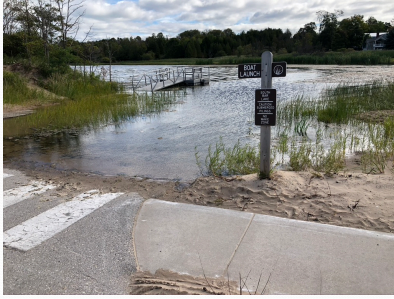
Public Boat Ramp Unusable South Bar Lake Sep 7, 2020
