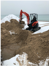
Trenching channel to Lake Michigan Jan 23, 2020
